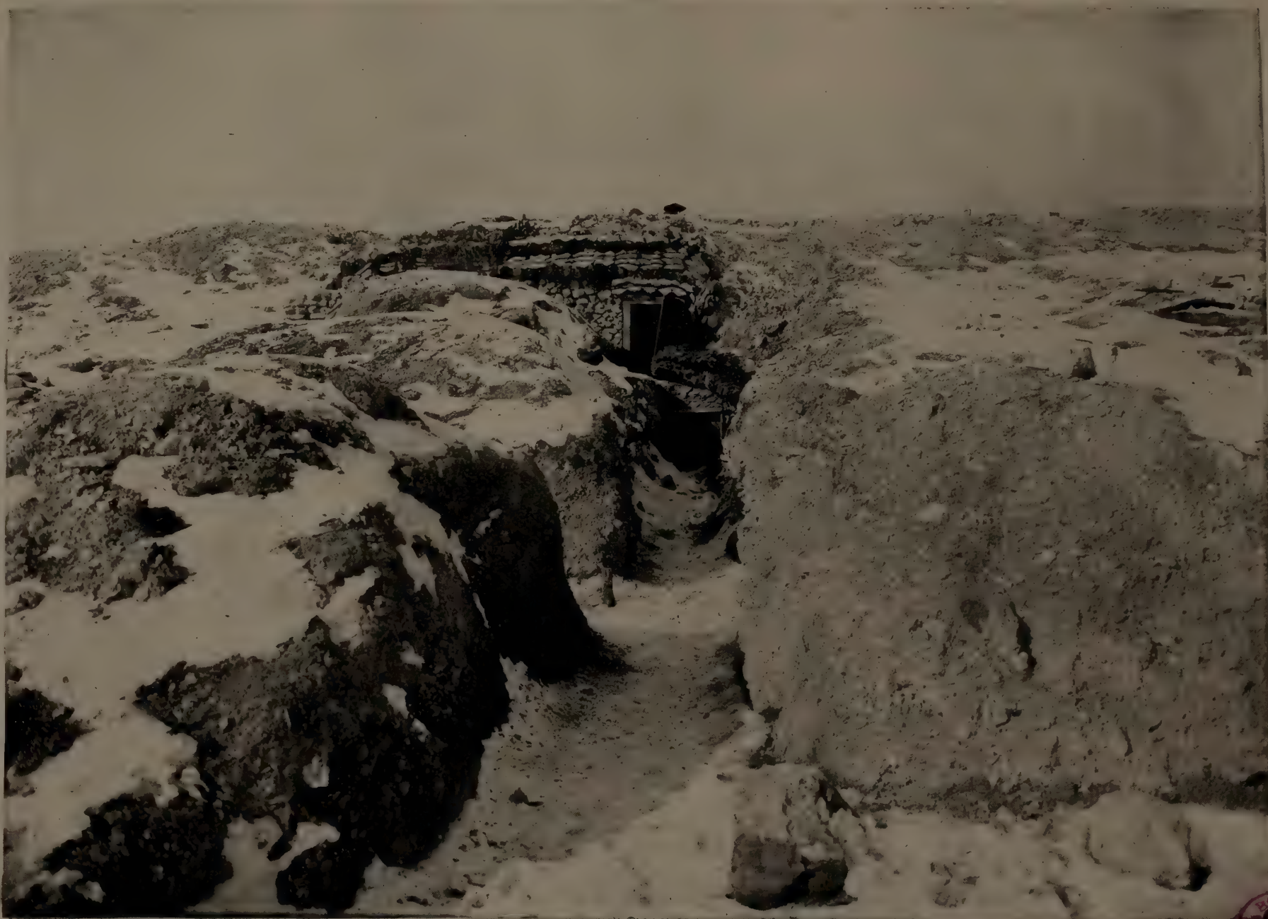
Winter scene in trench showing trench dugout
